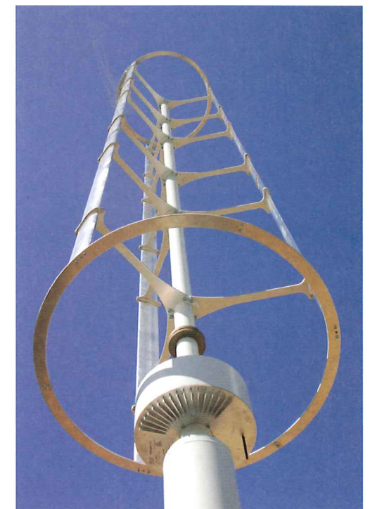
Spire-like wind turbines surround the perimeter of the parking lot and supply electricity to the LED luminaires on the canopy. The turbines offer artistic form and function, but added less than 1 percent to the project cost.
