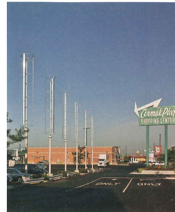
Spire-like wind turbines surround the perimeter of the parking lot and supply electricity to the LED luminaires on the canopy. The turbines offer artistic form and function, but added less than 1 percent to the project cost.
