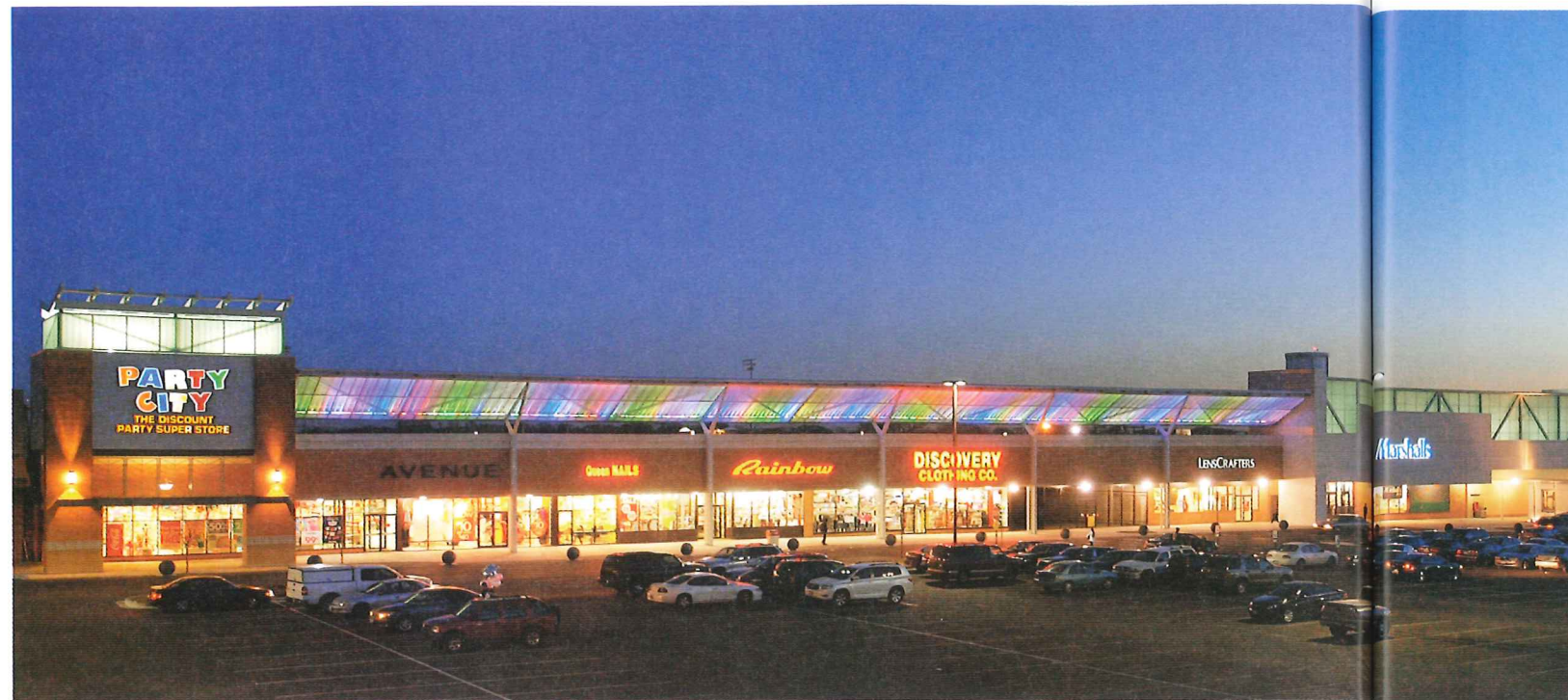
The luminaires are mounted inside the canopy, along the bottom edge. The canopy lighting changes colors, while the tower lighting (far left, above Party City) remains white. The objective was to use light to enhance the onsite customer experience and attract drivers passing by.
